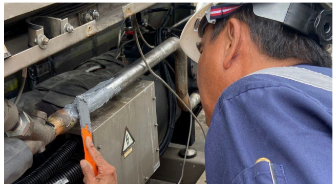
Belzona Epoxy Coating Supply & Application
